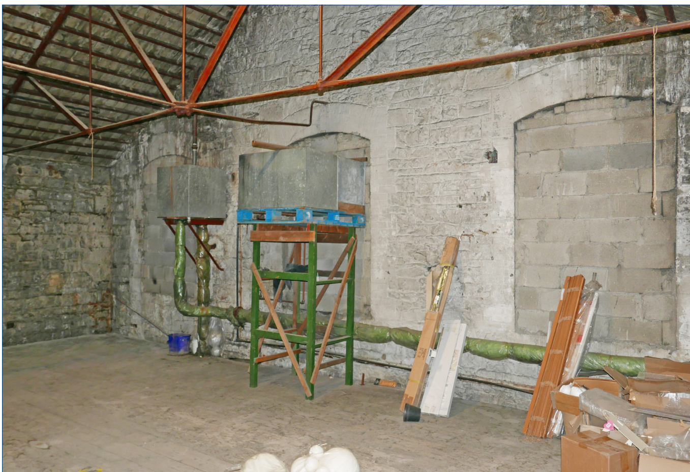
Large gabled building • upper floor • space at the north end of the building, looking north west.
