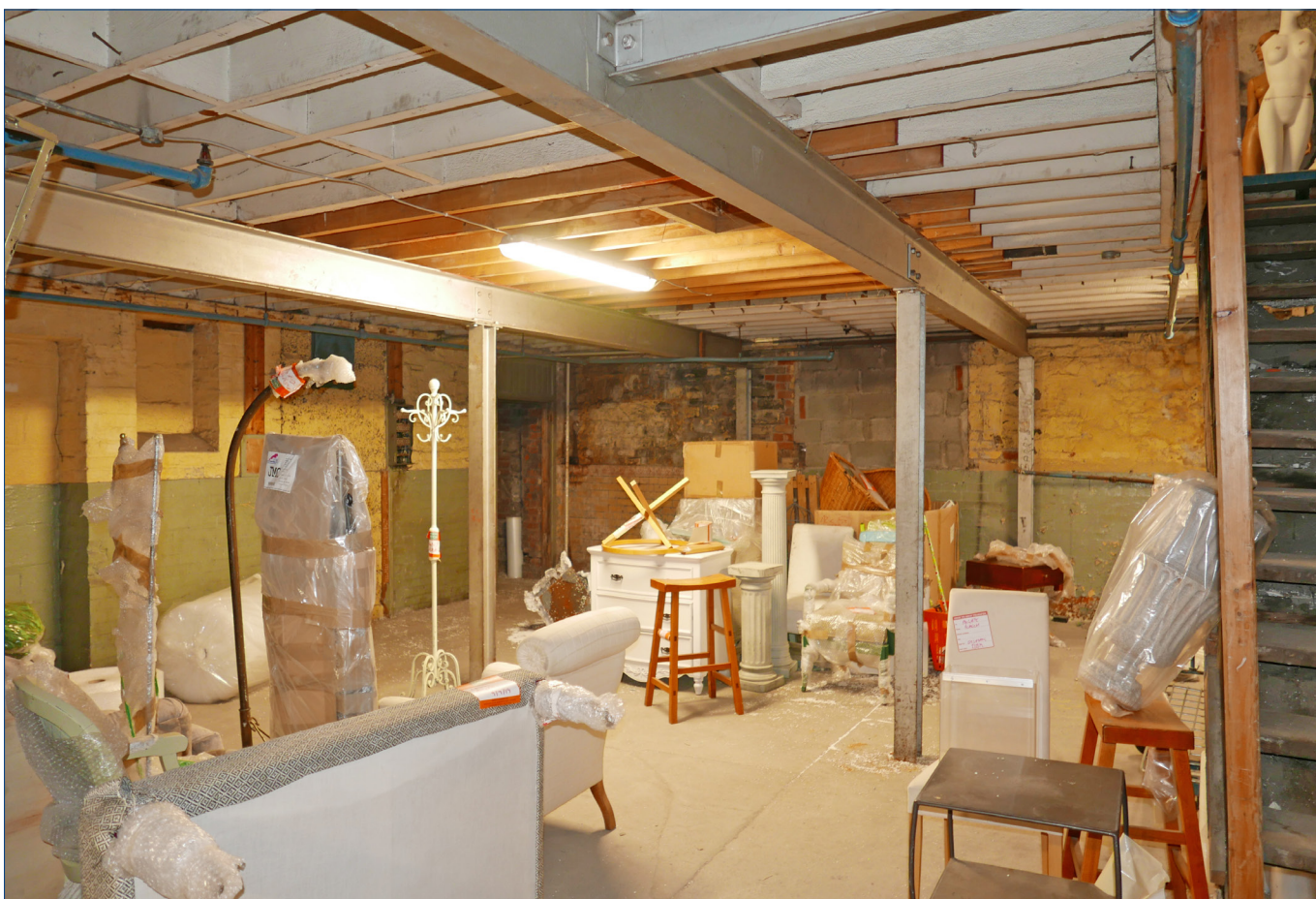
Small gabled building • Ground floor looking south east.
