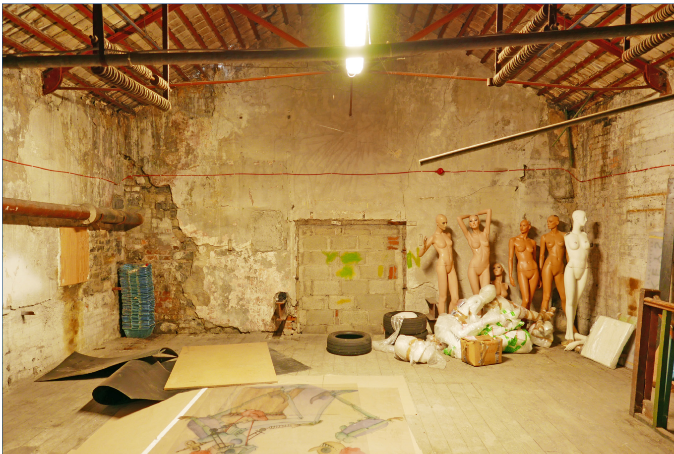
Small gabled building • Upper floor looking south.
