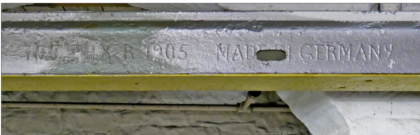
'105 PHX R 1905 Made in Germany' marked on a length of tram track that forms part of a mezzanine structure near the south wall of the Warehouse. It is possible that the mezzanine was built during the time the building was a munitions factory, making shells to fire at the Germans.
