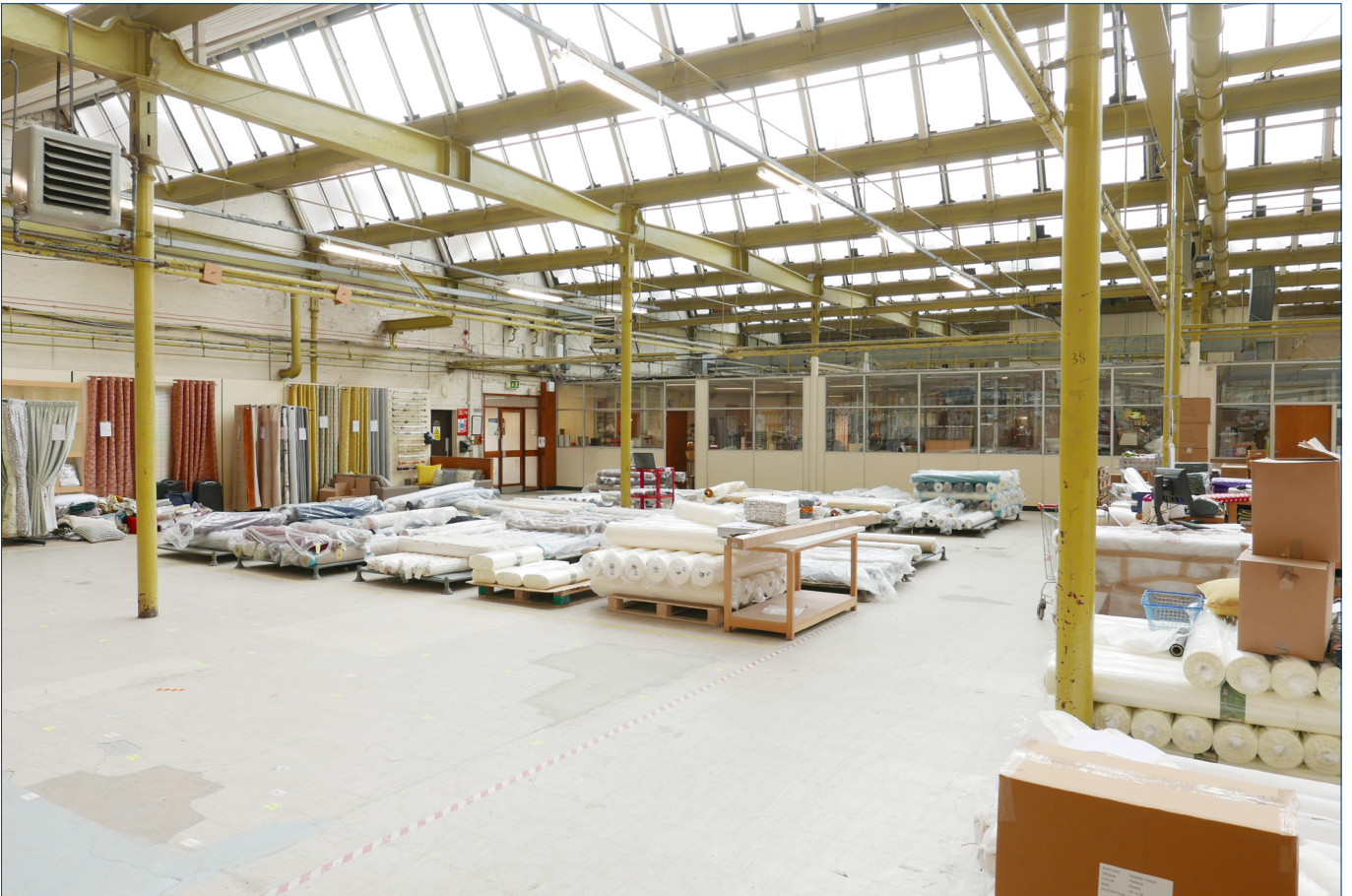
View in the Warehouse looking towards the north west corner. The 24 foot cast iron beams bear the name 'Courtney Stephens & Bailey'. These beams in turn support cast iron gutters spanning 12 feet that support the 'northlight' roof. It has not been possible to establish the origin of the columns supporting the roof beams.
