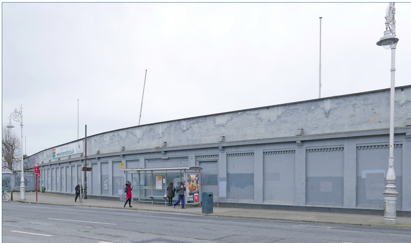
The curved wall of the warehouse on the south side of Parkgate Street. The wall is brick with brick piers, it was built in the 1880s
