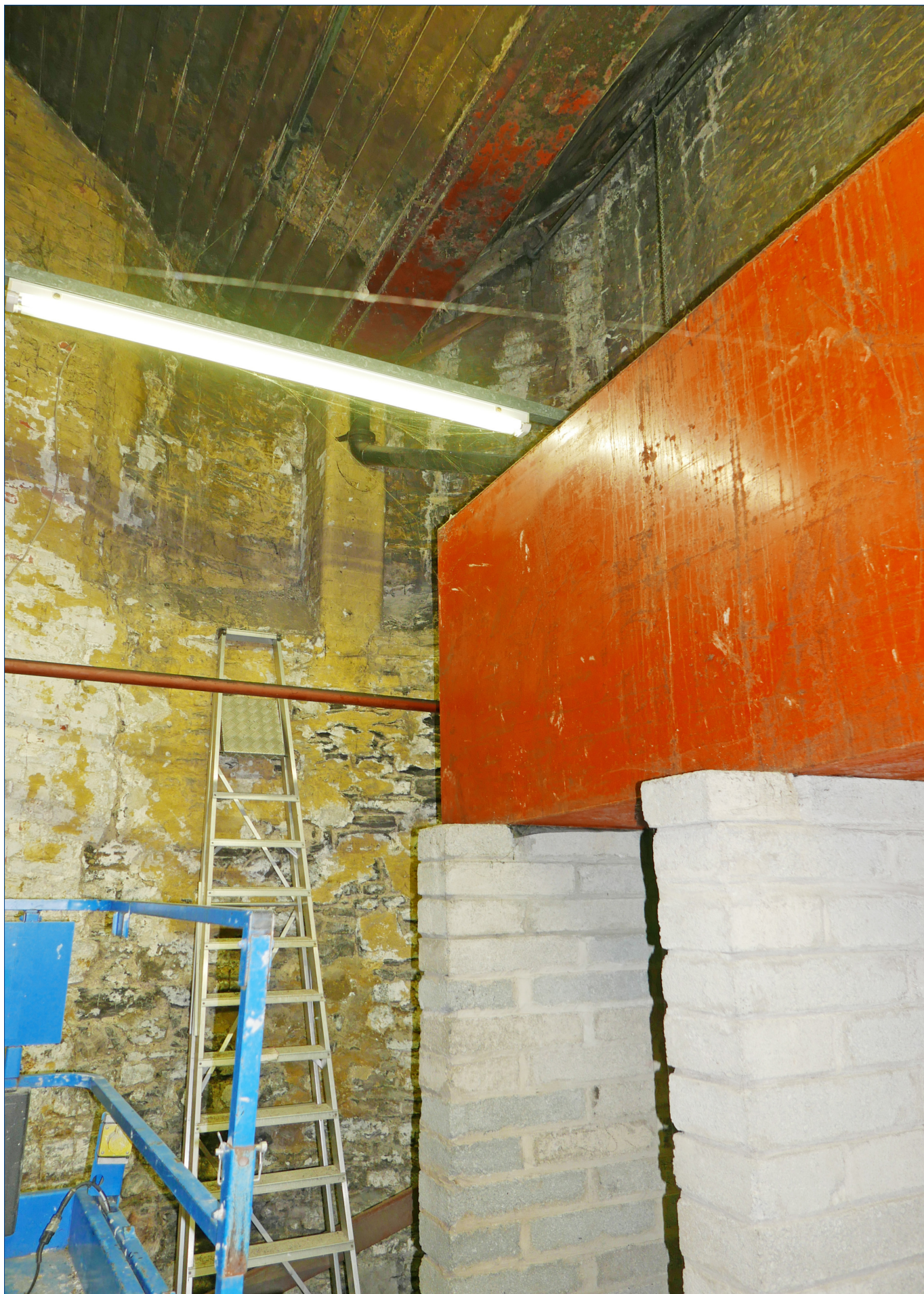
Interior of the Turret looking east. It will be noted, that for most of its height, the inner face of the wall of the Turret does not follow the curved line of the outside face. The inside face may have been built up in the 1880s in order to support the cast iron gutter carrying the roof of the Warehouse into the curve.
